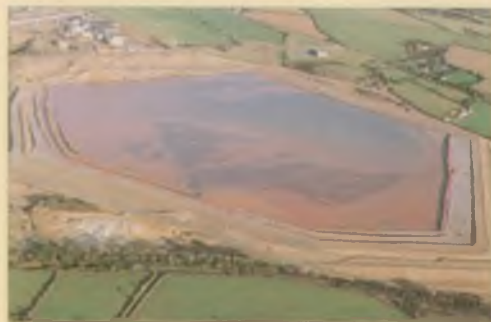
The metalliferous sediment settles into the Clemow's Valley Tailings Dam which is designed to store mine tailings arising from milling operations carried out on the site.
