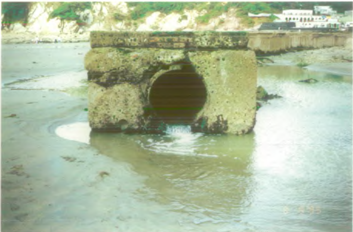
Plate 2. The Millendreath Stream culvert discharge onto Millendreath Beach at low water.
