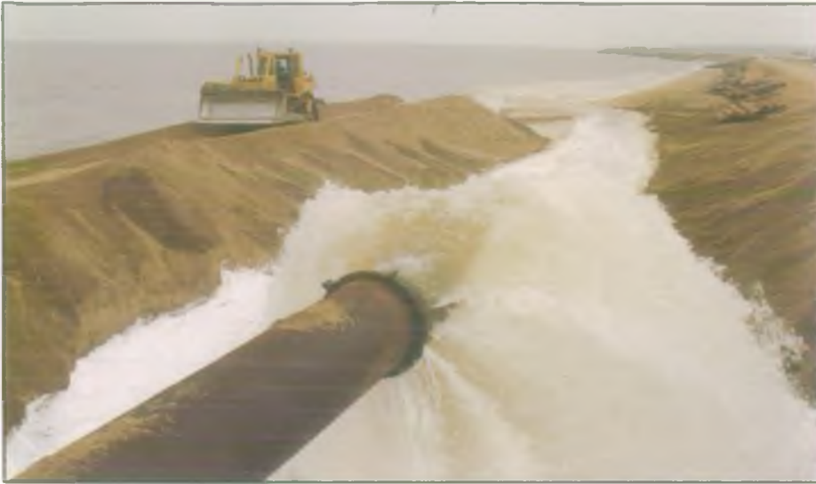
Heacham beach recharge in progress.
