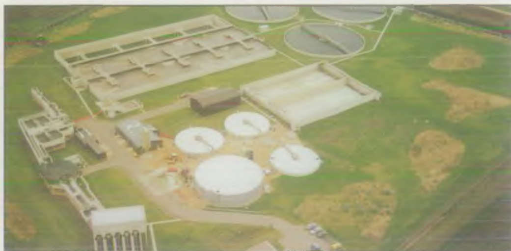
Flag Fen Sewage Treatment Works
