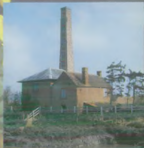
Westonzoyland Pumping Station, an early steam driven pump. Photo: Geoff Roberts, Somerset County Council.
