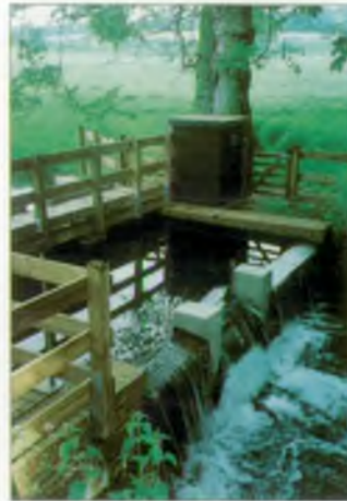
River flow measurement station upstream of Shardeloes Lake.
