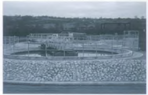
Ashbourne Sewage Treatment Works
