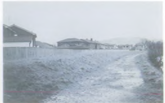
Houses at Ynysddu with flood protection
