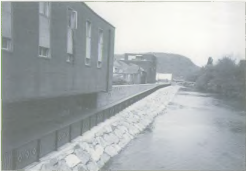
Flood defences on the River Taff in Pontypridd
