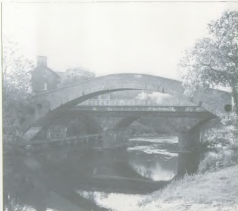
Pack Horse Bridge in Pontypridd
