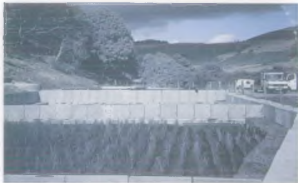
Peledda Mine Water Treatment Project
