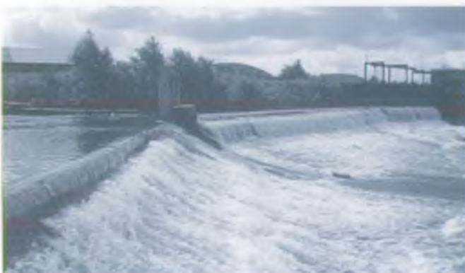
Afan Docks Weir
