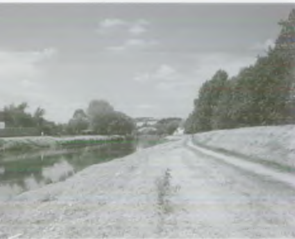
River Irwell, adjacent to Littleton Road Playing Fields
