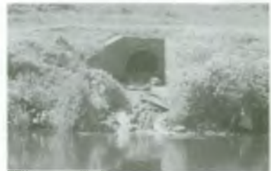
Outlet pipe, River Irwell
