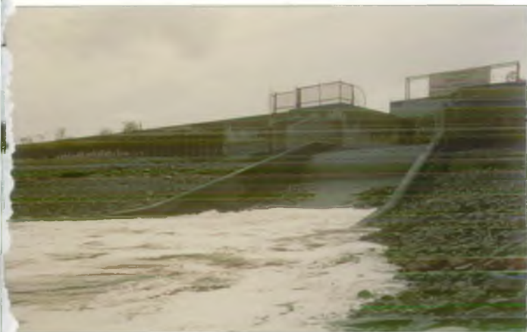
Beckton sewage treatment works outfall
