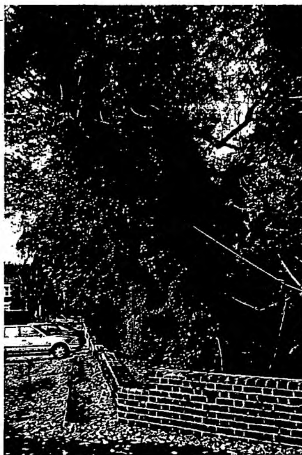
Fig. 3. Flood wall at Pound Mill
