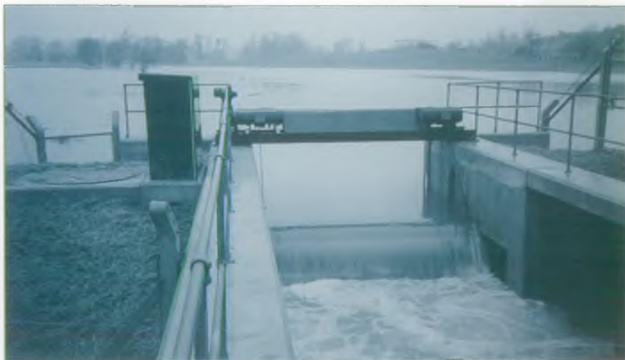
Part of A45 Flood Alleviation Scheme, R. Gipping, Stowmarket.
