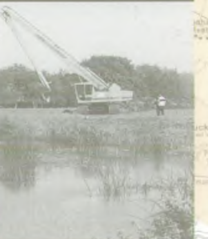
Channel maintenance, R. Beult
