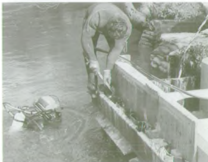
Fish pass construction
