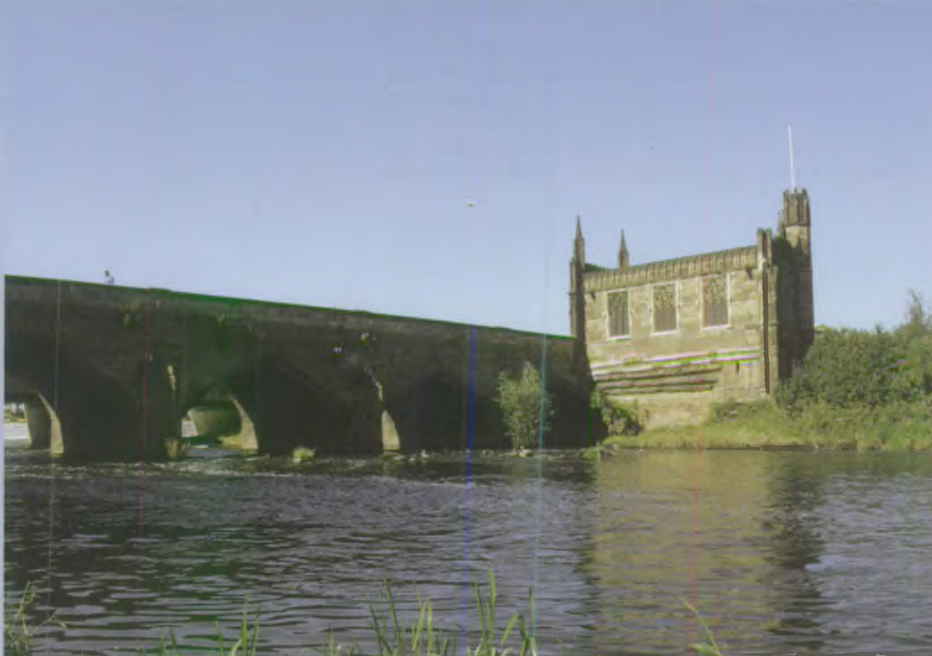
River Calder at Chanty Bridge, Wakefield
