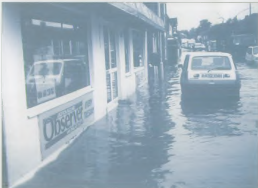
Flooding at Leighton Buzzard, September 1992
