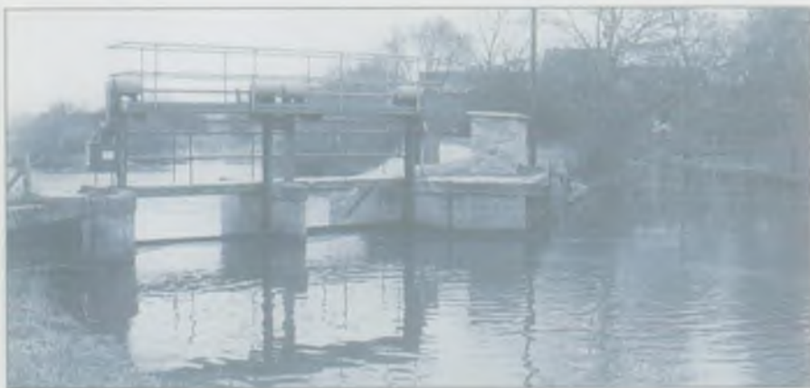
Control structure, River Ouse at Turvey
