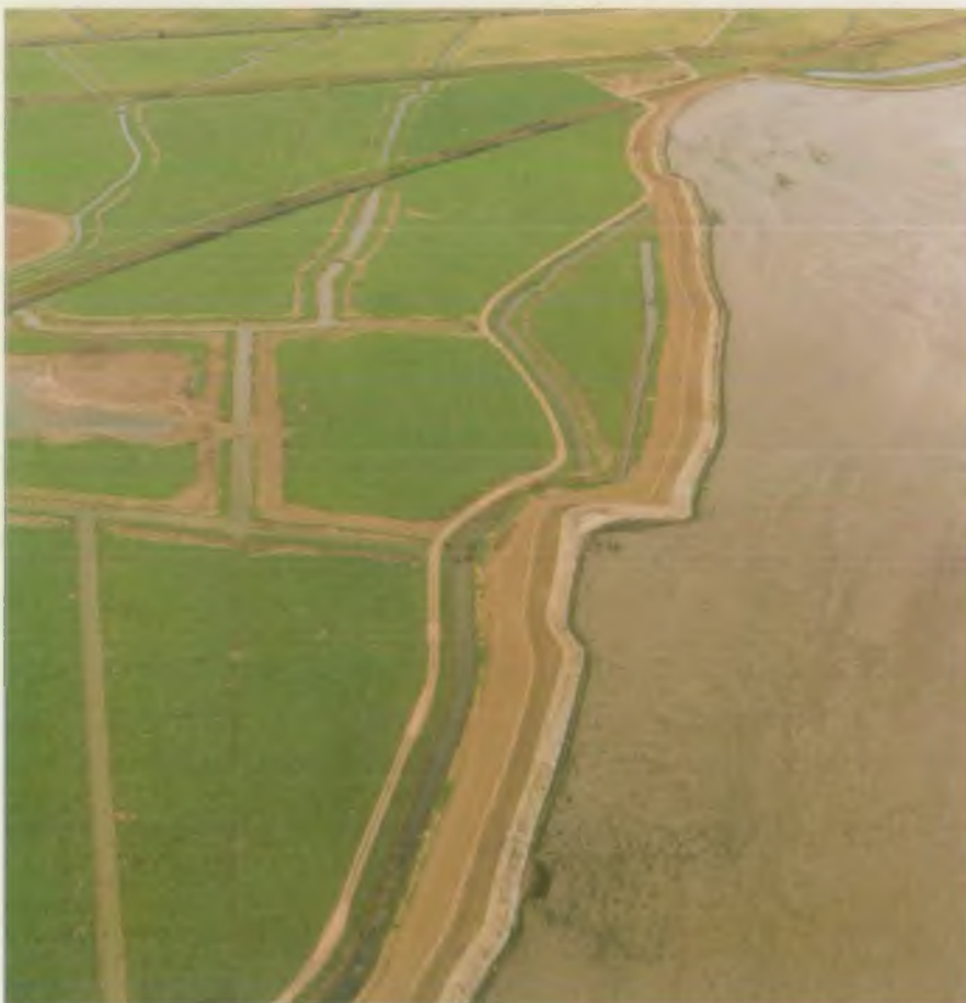
Above left: Works at Breydon Outfall Pumping Station
