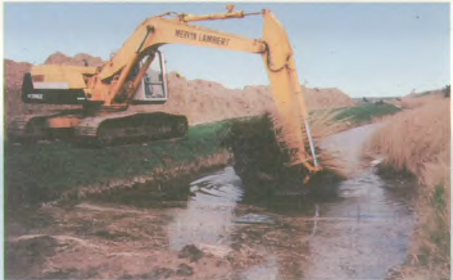
Right: Works to Soke Dyke at Ashtree Farm, River Yare
