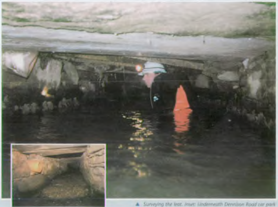
▲ Surveying the leat. Inset: Underneath Demisson Road car park
