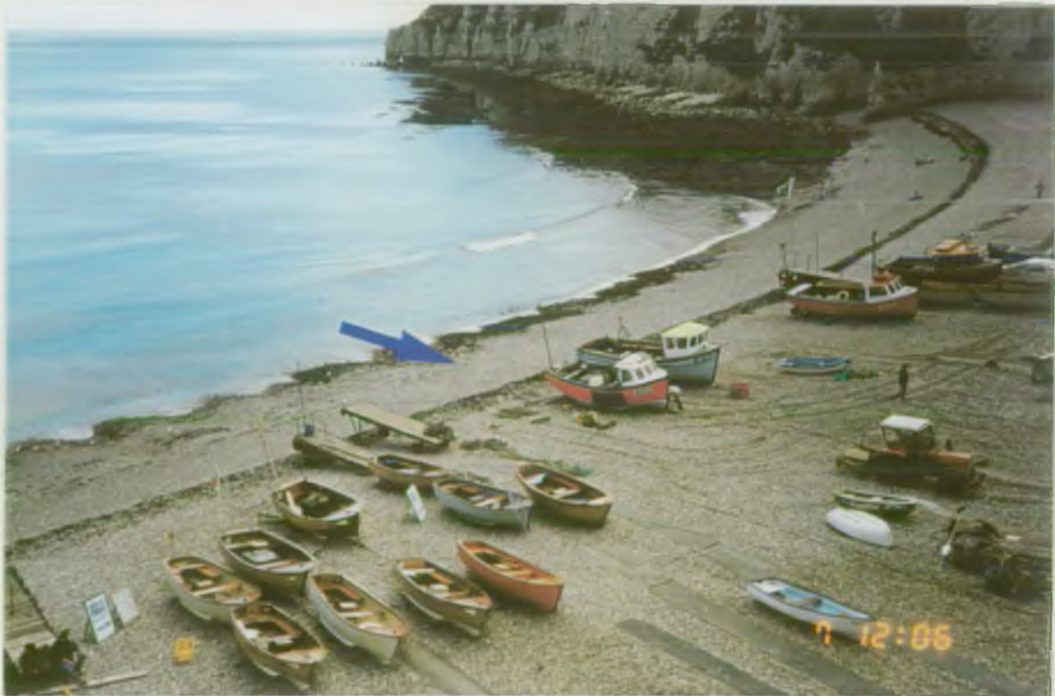
Photograph 6 Pipe discharge point
