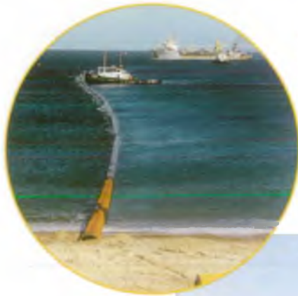
Beach recharge pipeline being positioned before sinking to the sea bed.
