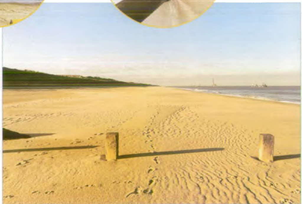
Completed section of beach recharge. South of sea Piling.
