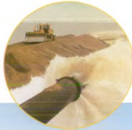
Beach recharge work in progress
