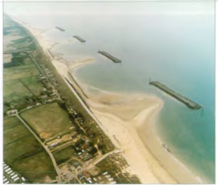
View of reefs completed in the first stage of defence works.
