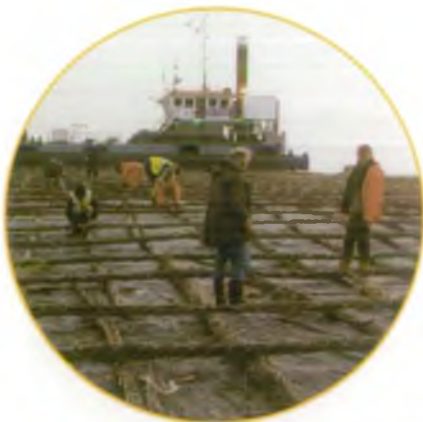
Construction and placing of reef materials
