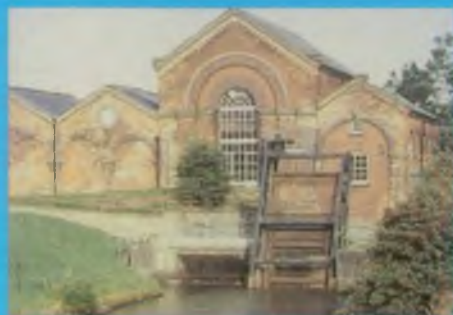
Dirtiness pumping station, on the North Level Engine Drain
