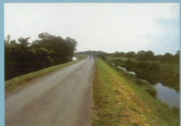
The North Level Engine Drain is now clear of Australian Stonecrop
