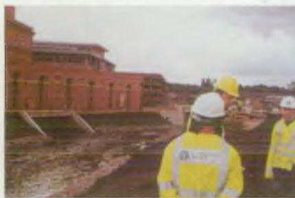
Kidderminster Town Centre flood alleviation scheme under construction
