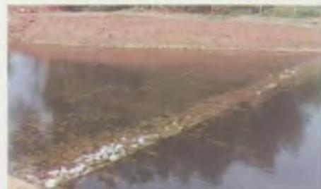
*A rock sill has been installed to maintain shallow water levels in the sediment filter to prevent the reedbeds from drying out*
