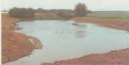
*New sediment filter slows down the flow of the River Eye to allow deposition of silt before the river enters the SSSI near Ham Bridge*
