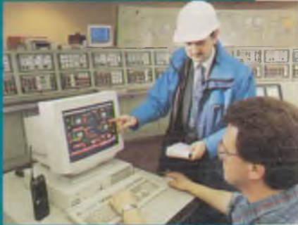
Inspection of process control systems at gas treatment facility
