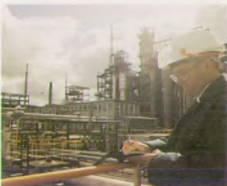
Major chemical installations are highly complex and need detailed assessment to prevent or minimise their emissions
