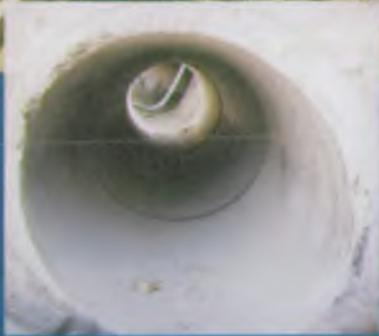
▲ The new entry pipe into the old culvert which discharges outside the harbour.
