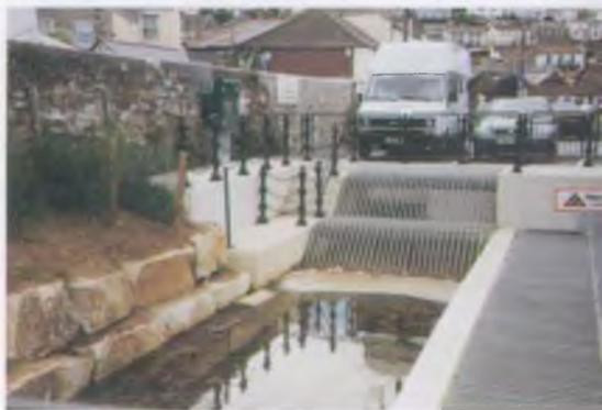
▲ The completed combined inlet structure with angled screens (pipe to old outfall in centre, new culvert entrance under screen on right).
