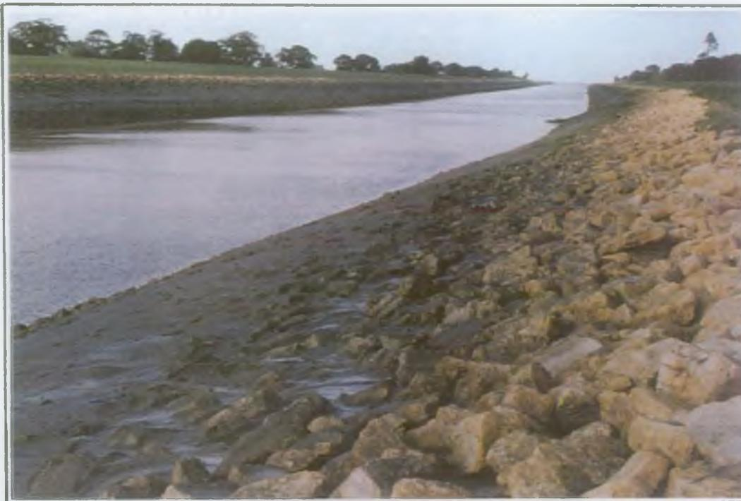
The installation of a 115,000 tonnes of machine placed stone toe and revetment to protect 4.2 km of flood defences.
