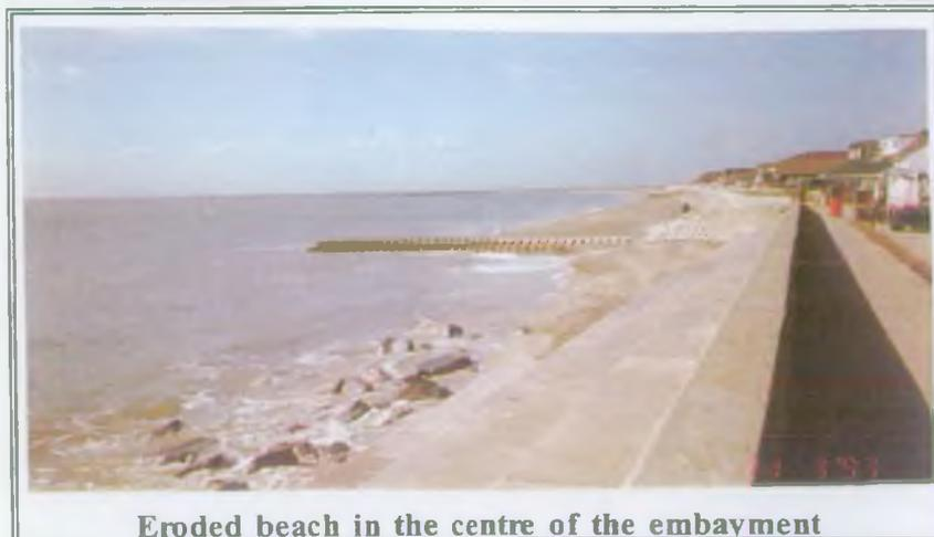
In the 1980's major work was carried out along this frontage when rock 'fishtail' breakwaters and beach recharge were constructed. Since the completion of those works, the beach has developed embayments with substantial deposit behind the breakwaters, yet eroding areas in the centre of each embayment.
