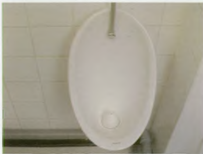
Conversion of urinals to waterless operation at the Agency's Lichfield offices, in the drive to reduce water consumption
