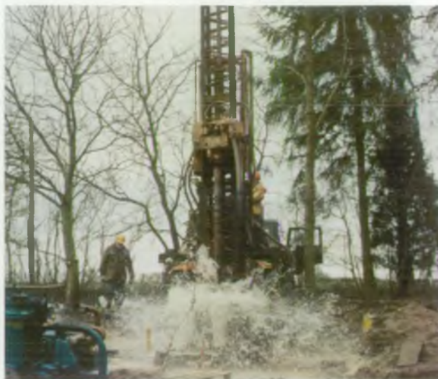
Drilling of a Shropshire Groundwater Scheme borehole to provide additional flow regulation support for the River Severn
