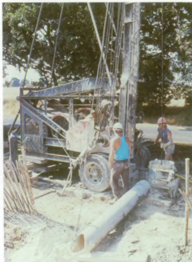
A drilling rig engaged in borehole construction at Swanton Morley
