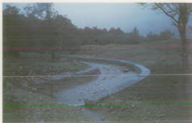
Gabion reinforcements used to restrain the active channel of a mountain valley river (above) - such reinforcements often fail, for example, on the River Swale, Yorkshire (below)
