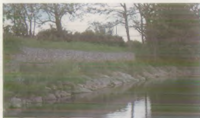
Gabion reinforcement and, on lower bank, rip-rap
