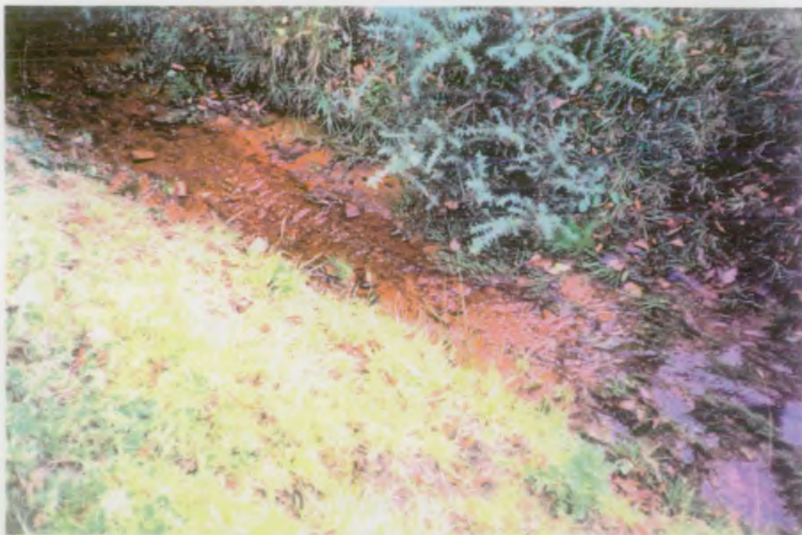
Iron ochre deposits in the land drainage ditch.
