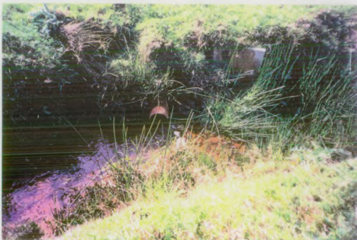
Land drain entering the land drainage ditch.
