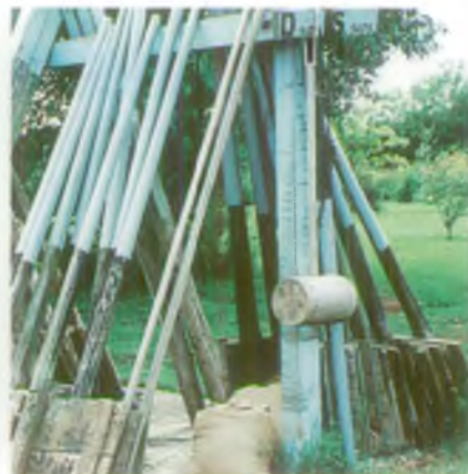
PLATE 9 Paddle rack for paddle and rymer weir in the Upper Thames.
