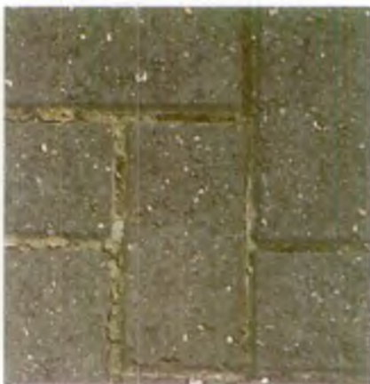
PLATE 19 Concrete block paviors - charcoal grey. Two years after laying.
