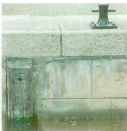
PLATE 11 Stone lock chamber wall with granite copings at Iffley Lock.
