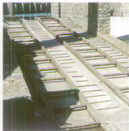
PLATE 14 Boat roller ramps at Molesey.
