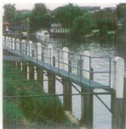
PLATE 6 Galvanised steel guard rails against timber piles with white flashes.
