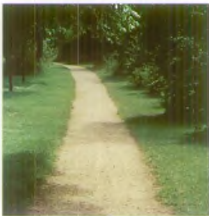
PLATE 23 Crushed stone footpath without retaining timber edge.
