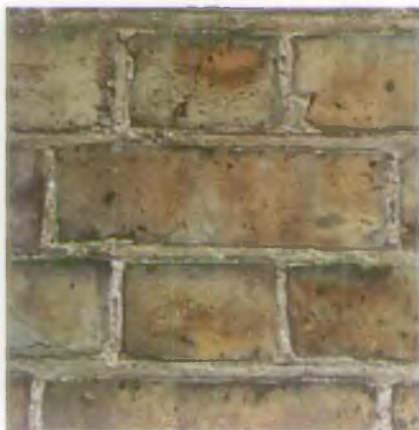
PLATE 21 London stock facing bricks with lime mortar.
