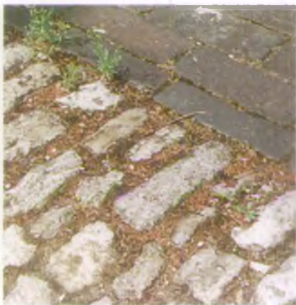
PLATE 22 Stone setts with blue brindle engineering bricks - mellowed with age.
