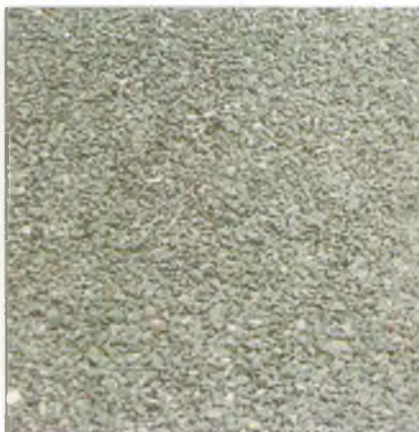
PLATE 18 Bound macadam - with granite chippings rolled into cut back bitumen.
