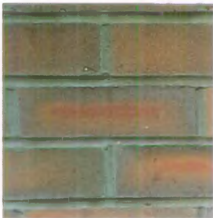
PLATE 20 Engineering quality red brindle facing bricks with cement/sand mortar.
