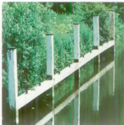
PLATE 8 Offshore timber lay-by in Buscot Reach.
