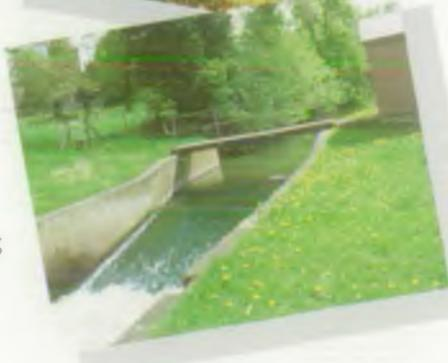
At gauging stations, because the processes of erosion and deposition continually change the shape of natural rivers, it is sometimes necessary to build stable structures such as weirs. A calculation is then used to convert the level of the river accurately into flow.
