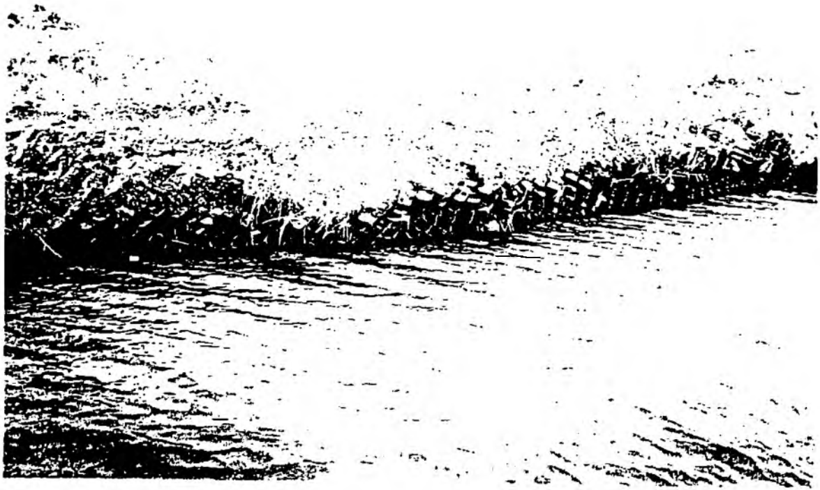
6.1 GEOWEB INSTALLED ON RIVER BANK
