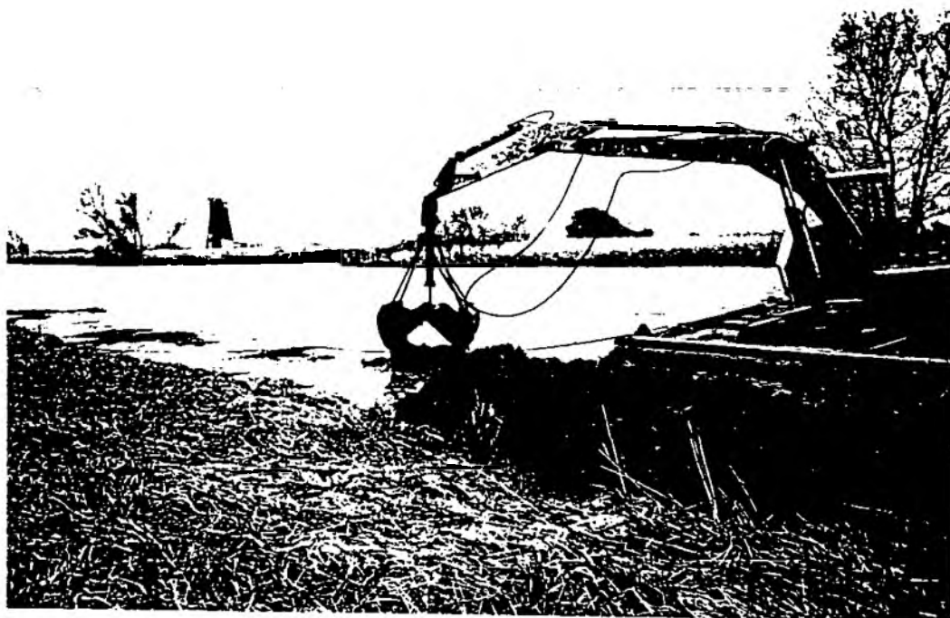
10.1 MATTRESS BEING BACKFILLED
