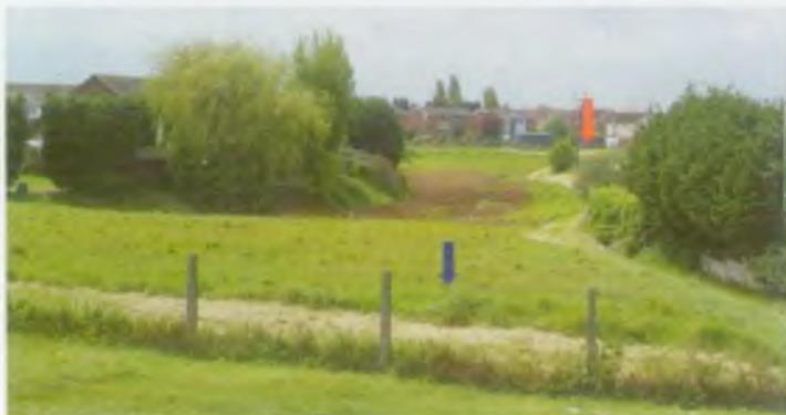
Site works at Croppenburg may involve moving the pumping station from its current location (the red arrow) to a location closer to the sea wall within Environment Agency owned land (approximately marked by the blue arrow)
