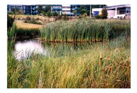
Plate 4. Vegetated balancing pond at Aztec West Business Park, near Bristol, with ecological features and aeration
