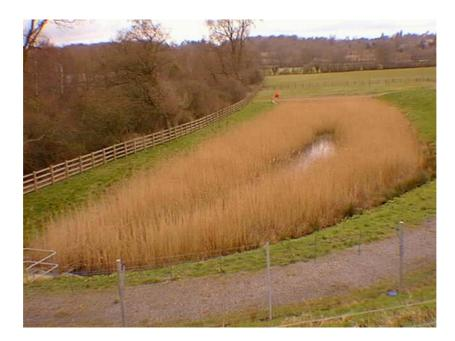
Plate 3. A constructed wetland within a commercial development in Milton Keynes, providing flood storage, pollutant treatment and aesthetic amenity value
