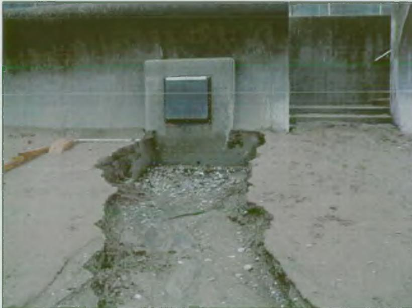
Plate 5, secured manhole on P4 discharge line showing tidal flap
