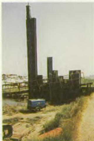
Driving steel sheet piling to form cofferdams, cut off walls etc.
