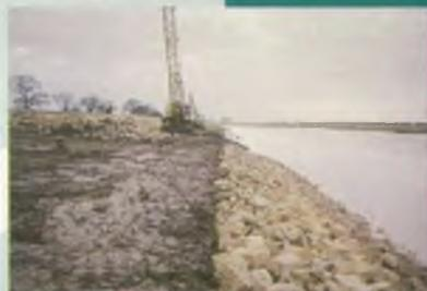
Stone revetment being replaced using a 22RB dragline to protect batters from erosion on tidal channels.
