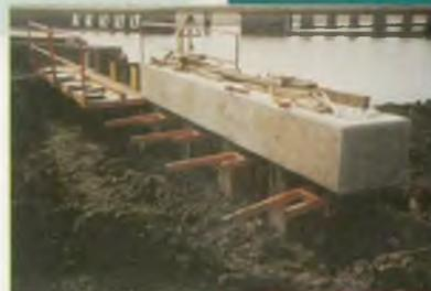
Casting reinforced concrete capping beams to steel sheet pile wall.
