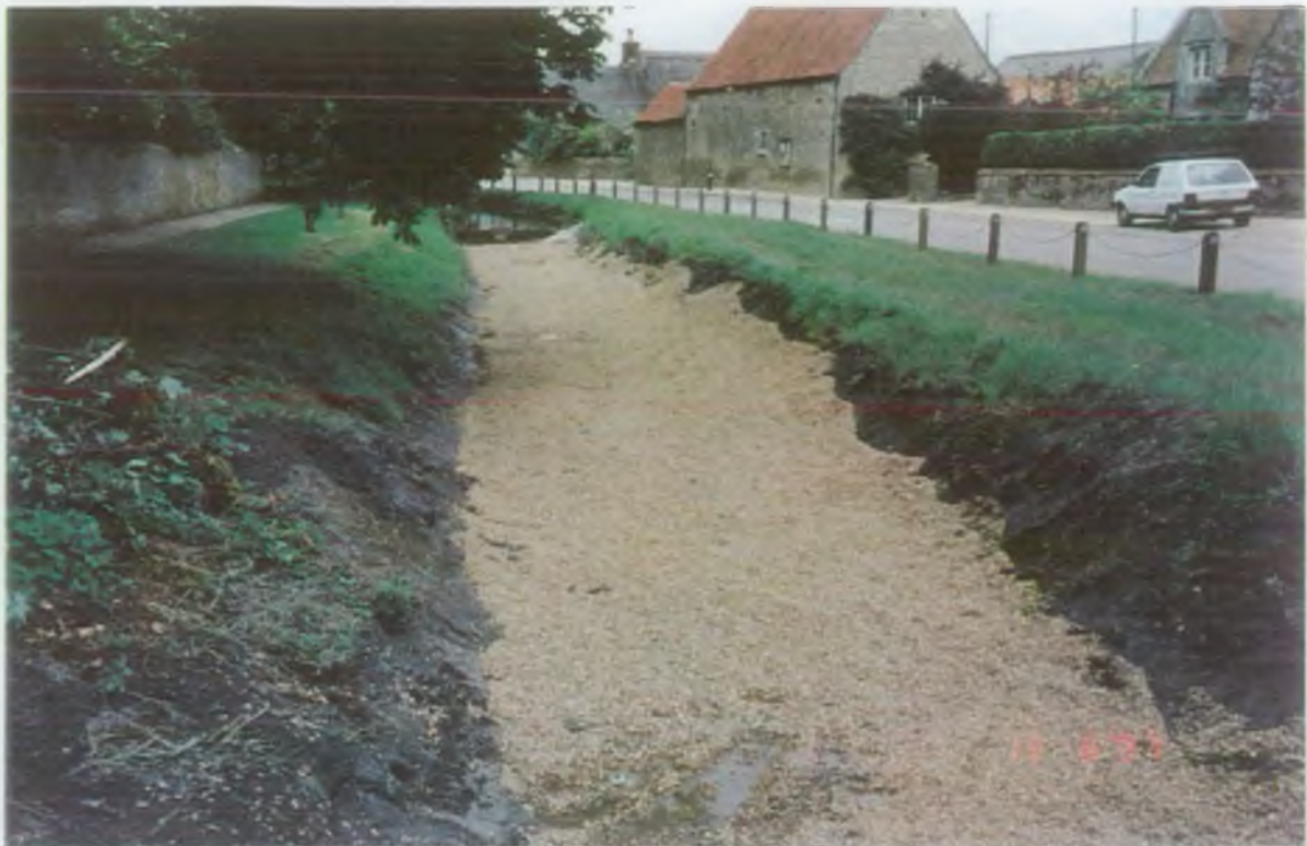
Formation of Gravel Bed, Alledge Brook - Grafton Underwood
