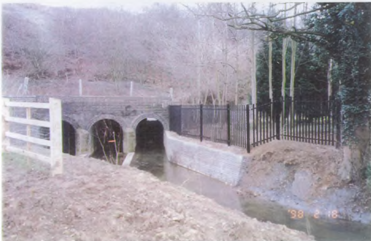
Completed Training Works to Railway Tunnels
