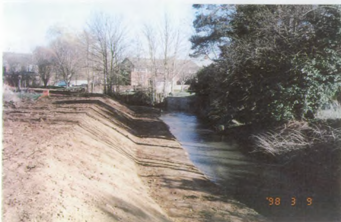
Channel Re-Sectioning
