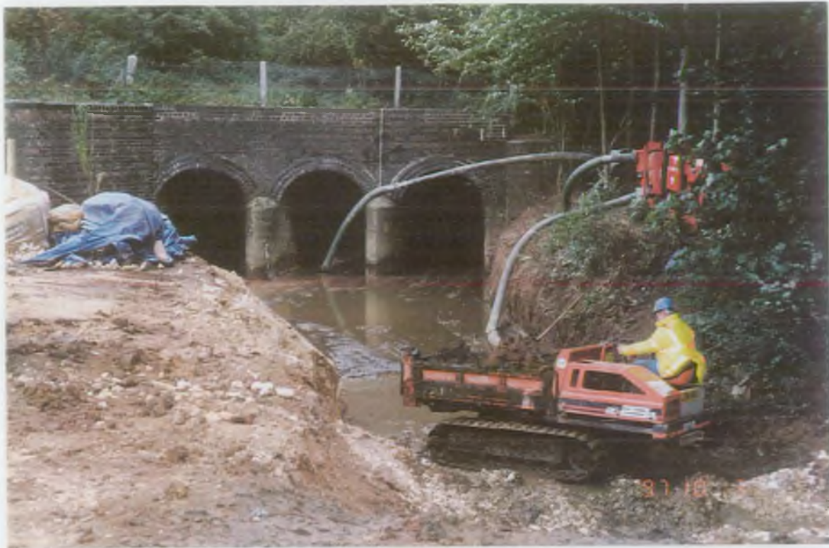
Improving Channel Alignment - Entry to Railway Tunnels
