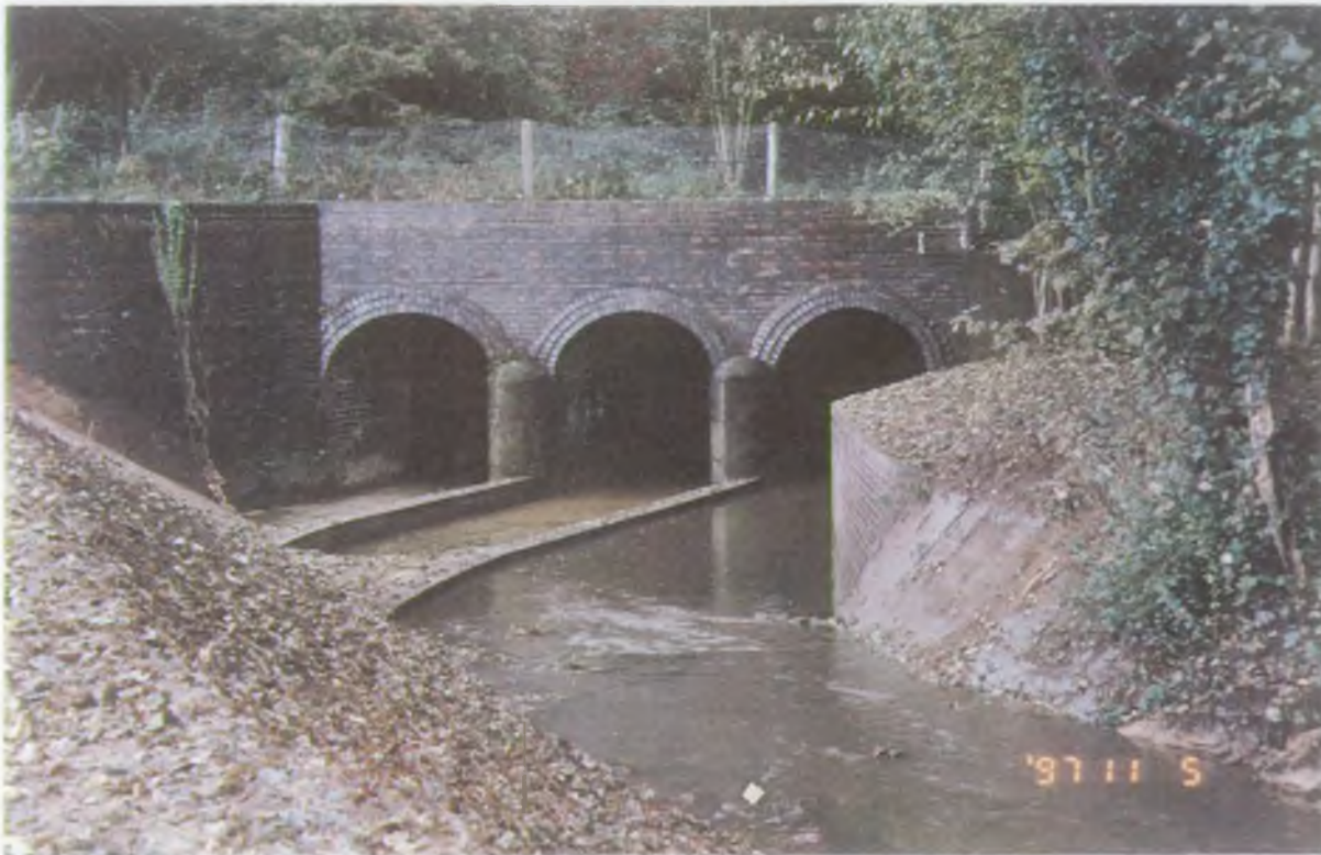
Training Works - Entry to Railway Tunnels
