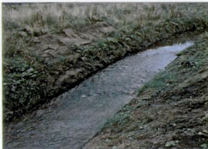
One of two gravel riffles installed on Brunstock Beck in 1999
