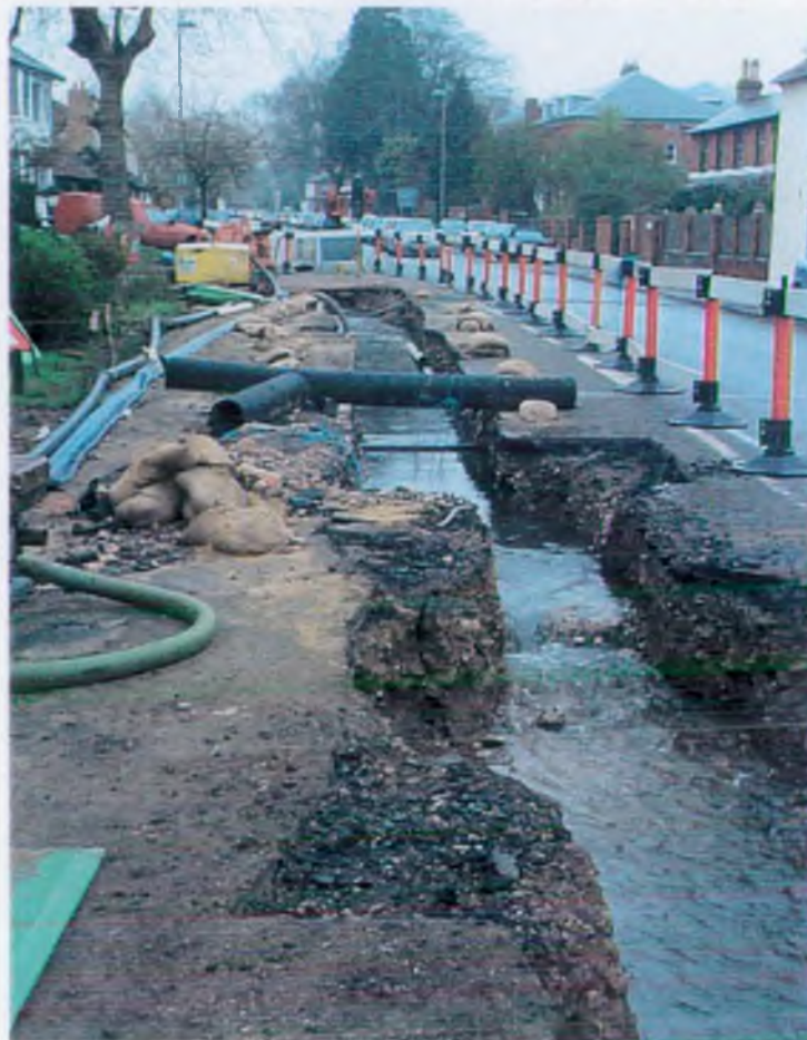
Figure 27: Renewing culverts under the A3130 in Henley to cope with the exceptional flow, 14/04/01.
