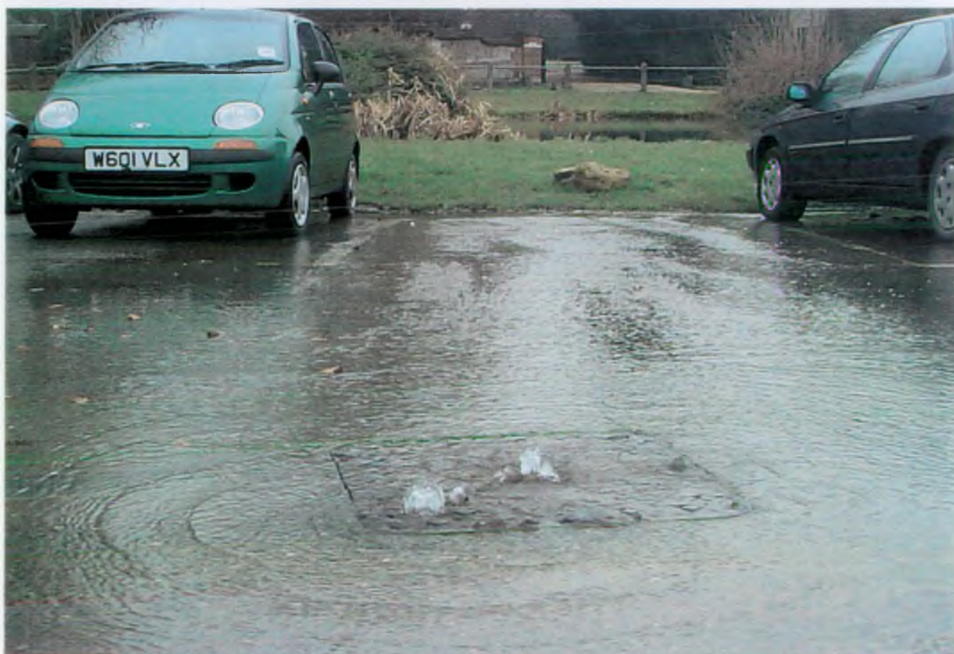
Figure 15: Groundwater surcharge of drains in Aldbourne SU 264 756
